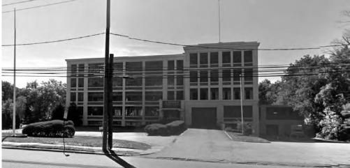
Description: This 4 story, 14 bay concrete pile is an "L" shaped plan with a flat roof and classical terra cotta detailing. Details on the exterior include brick faced reliefs and large, multi-pane industrial sash windows. Terra Cotta details are visible such as an entablature, pilaster strips at major columns and parapets at the roofline.
