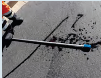
Wand used to loosen debris
