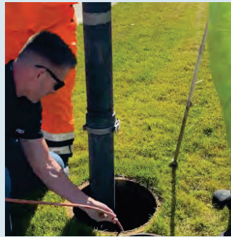
Vacuum removal of debris
