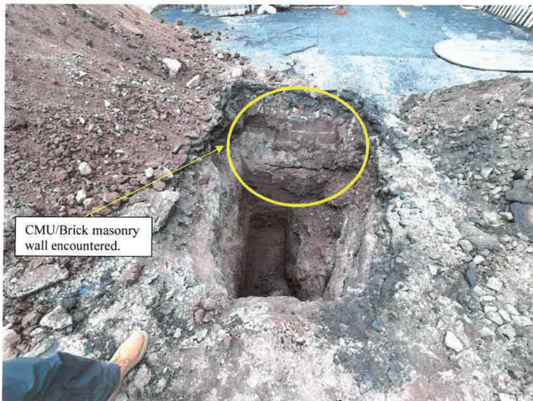
Test Pit Location – 01 (@ 11' – 0" depth)
