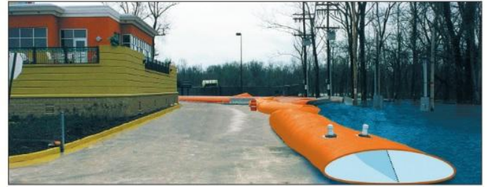
Figure 4-23. Three-foot-high water-filled temporary barrier protecting a structure in Tunica, MS (source: Hydrological Solutions, Inc.)
