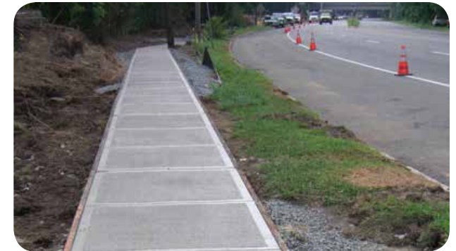
New sidewalk. Image: VTC
