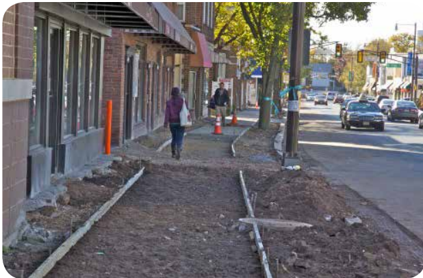
Sidewalk ready to be poured. Image: VTC
