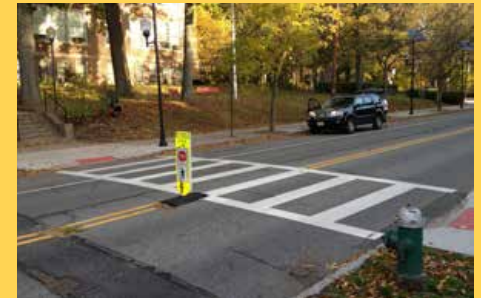
Newly painted high visibility, continental crosswalk and in-pavement “Stop for Pedestrians” crossing sign. Image: Arterial
