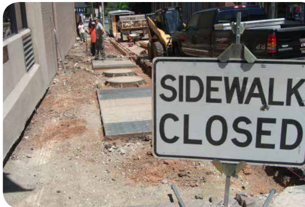
Sidewalk closed for repairs. Image: VTC
