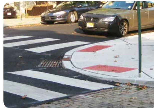
Intersections should have two perpendicular, ADA-compliant curb ramps per corner. Image: The RBA Group
