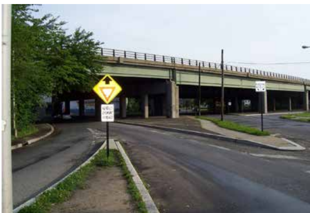
The crosswalks are unmarked and curb ramps absent at this ramp, located one block from an elementary school in Camden. Image: Cambridge Systematics
