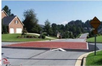
Raised intersections are good for locations with substantial pedestrian activity, areas where taking away parking spaces would be unacceptable or where locating humps in front of residential properties is a problem.
