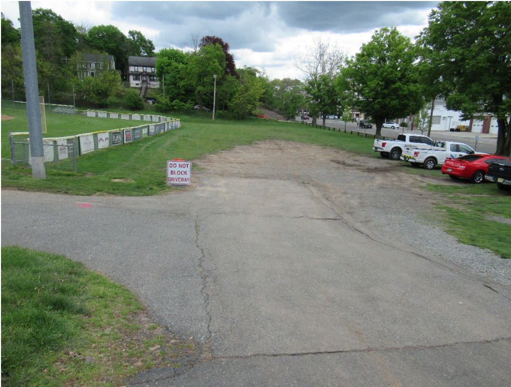
Photograph #1: Existing site public parking area
