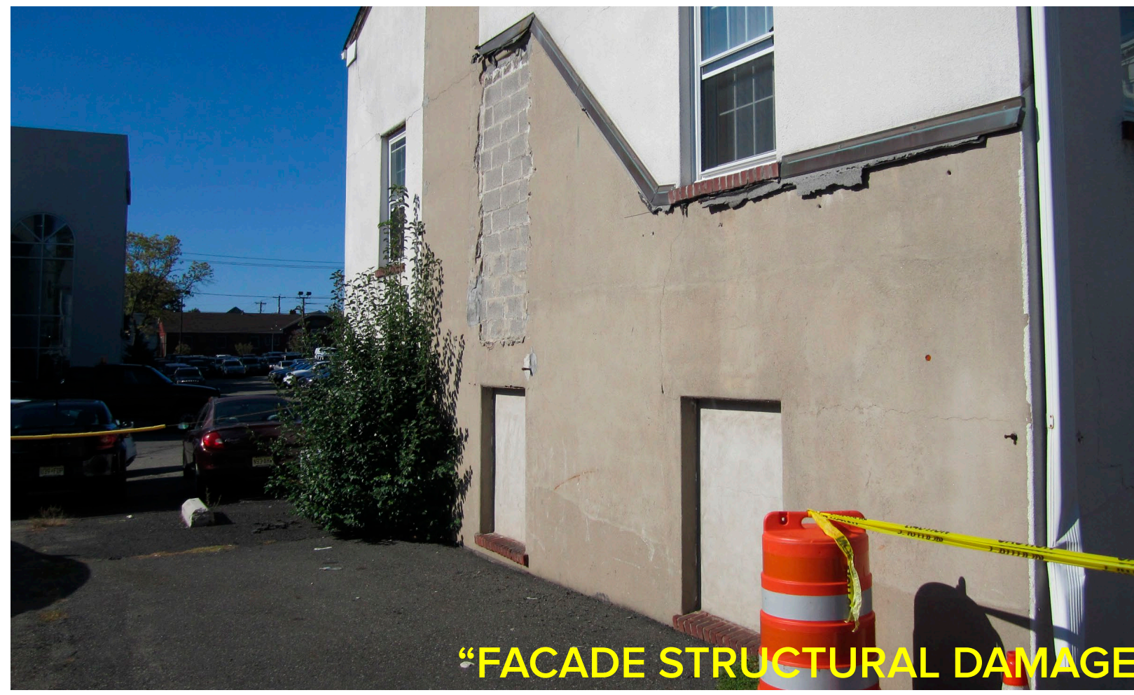
"WATER DAMAGE - STUCCO - CAN SEE DAYLIGHT"
