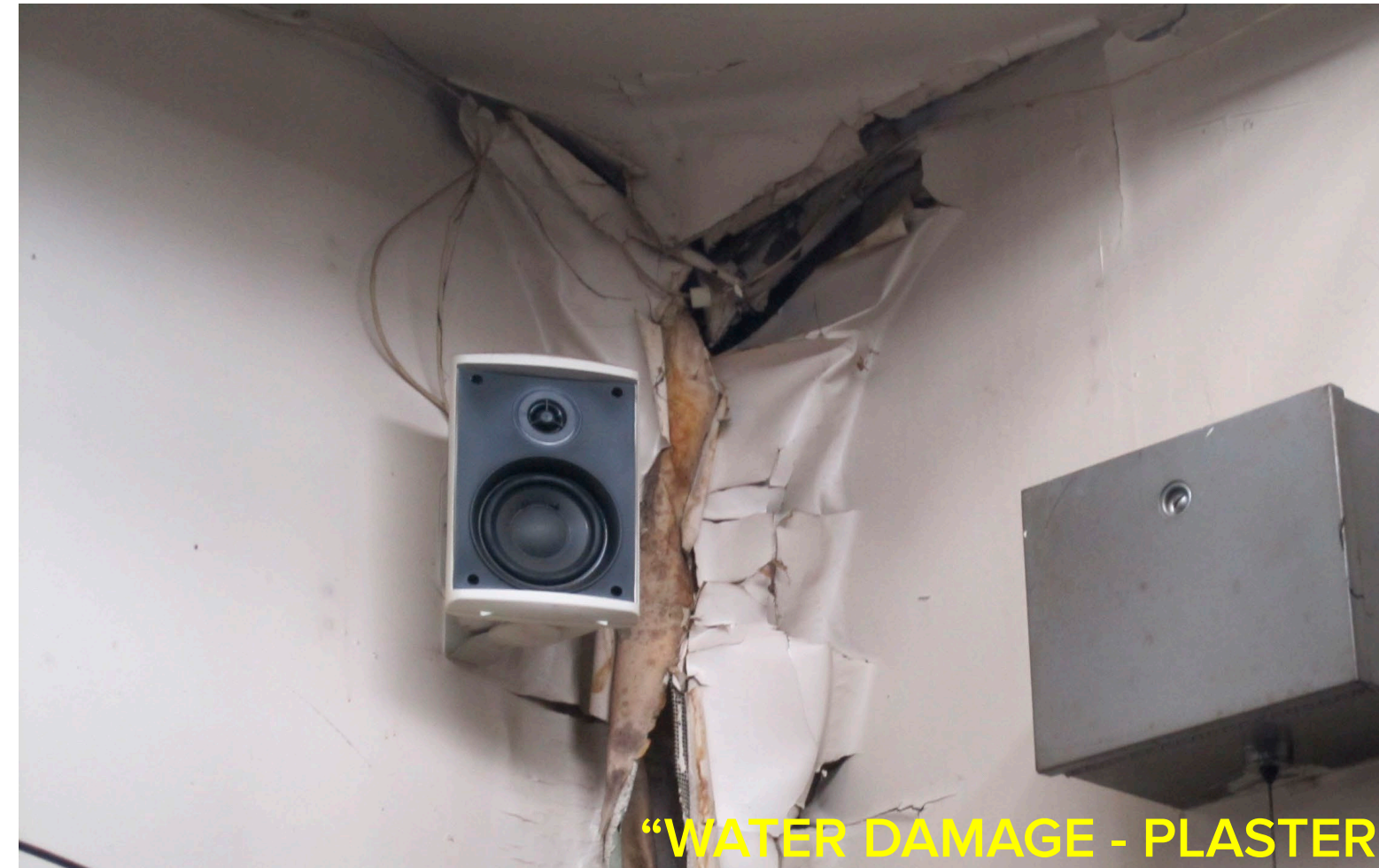
"WATER DAMAGE - PLASTER"
