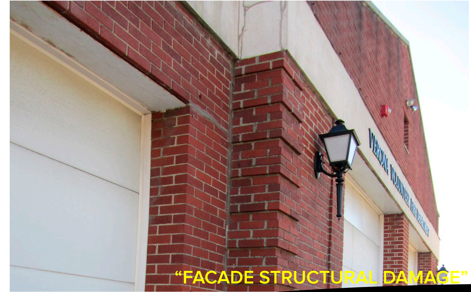
"STRUCTURAL SETTLEMENT CRACKING"
