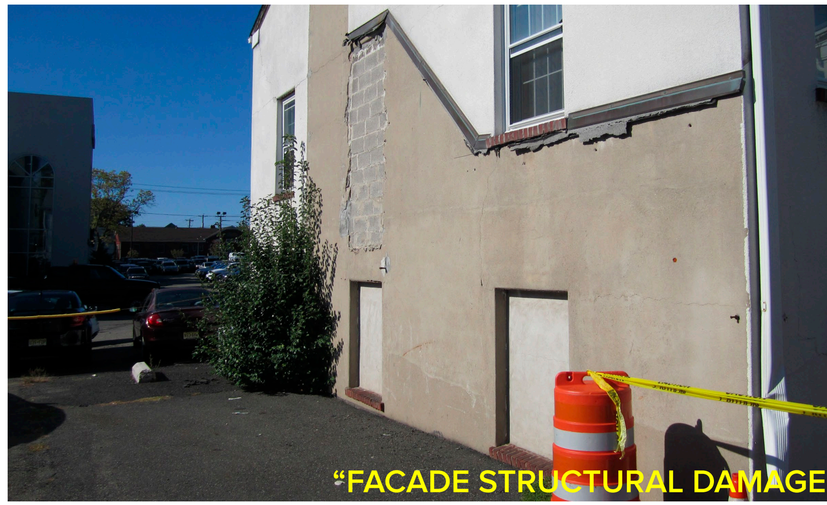
"WATER DAMAGE - STUCCO - CAN SEE DAYLIGHT"
