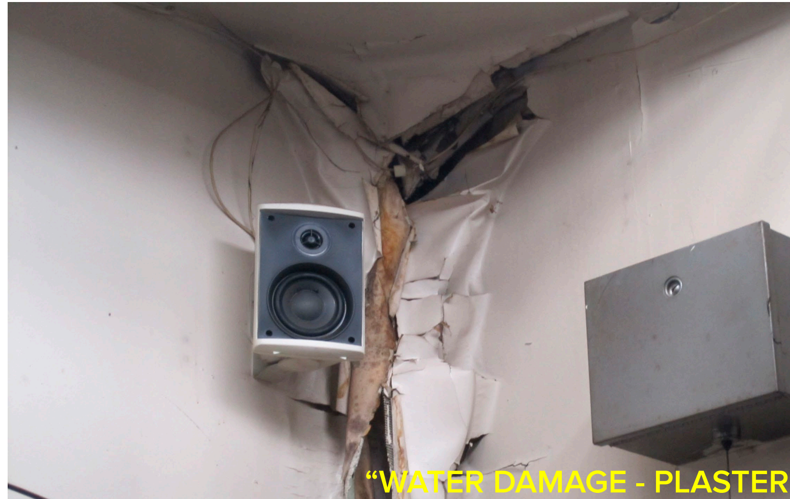
"WATER DAMAGE - PLASTER"
