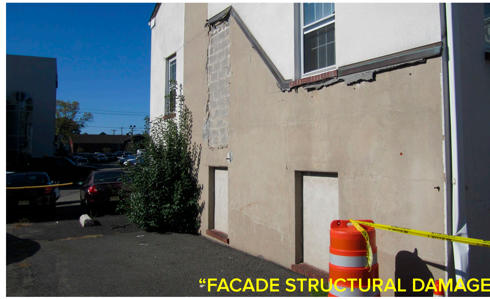
"WATER DAMAGE - STUCCO - CAN SEE DAYLIGHT"
