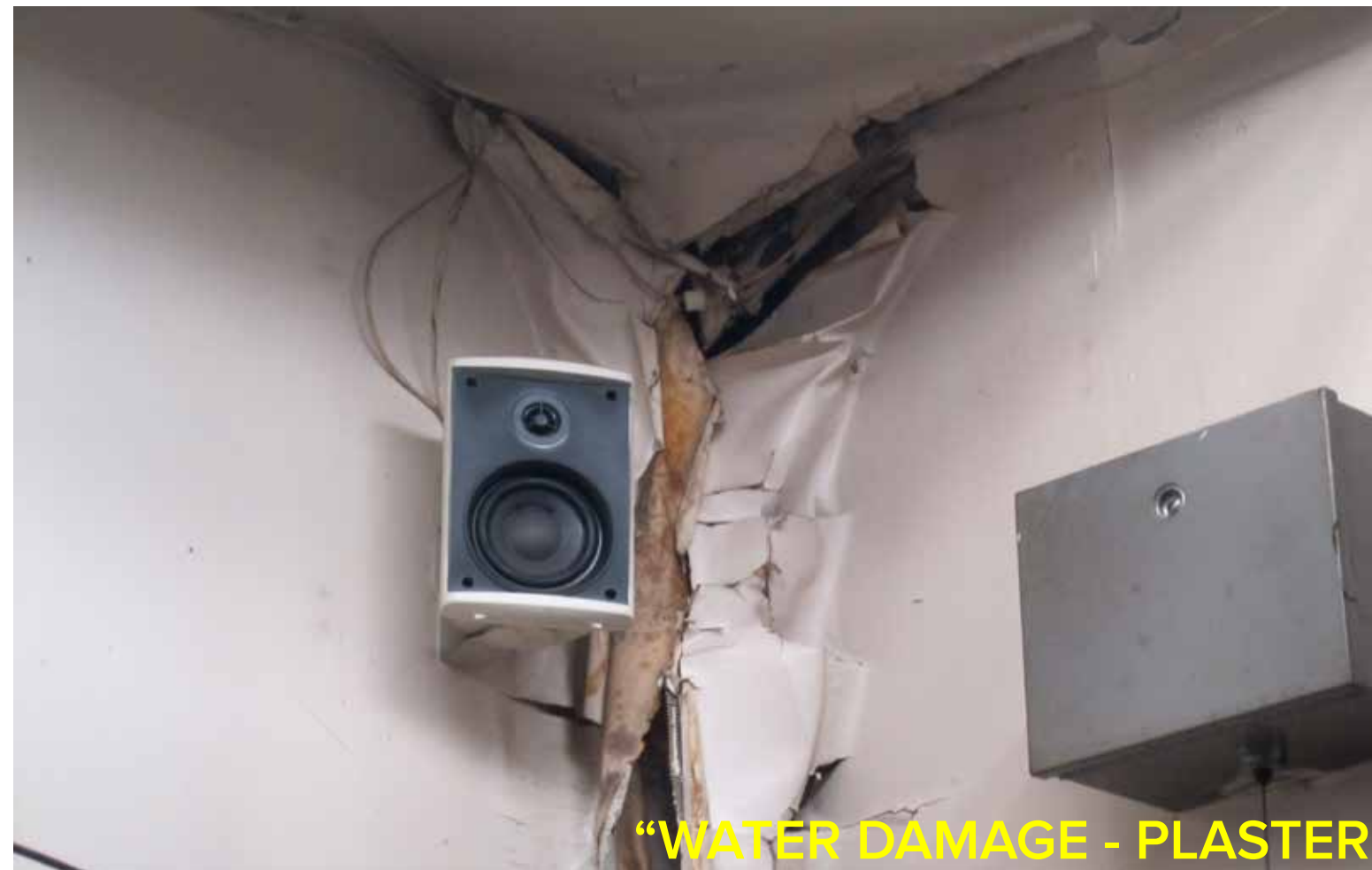
“WATER DAMAGE - PLASTER”
