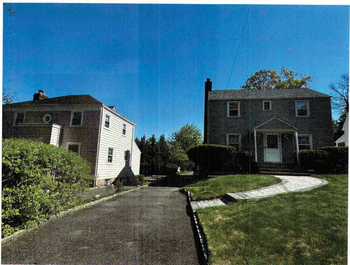
FRONT VIEW OF HOUSE AND NEIGHBOR TO THE RIGHT (FROM STREET)
