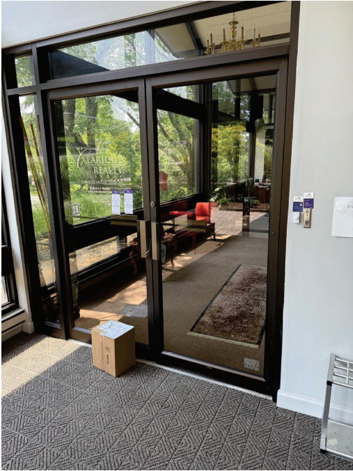
BUILDING LOBBY 321 ENTRANCE
