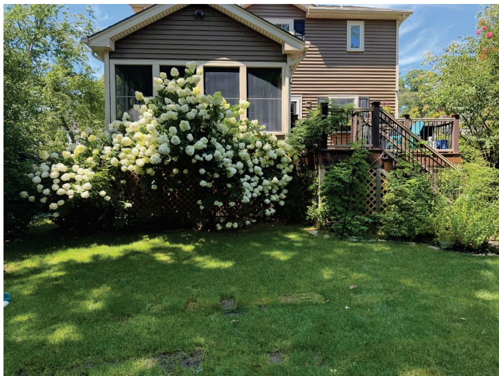
Photo 4 – View of the rear elevation of the dwelling and rear deck.
