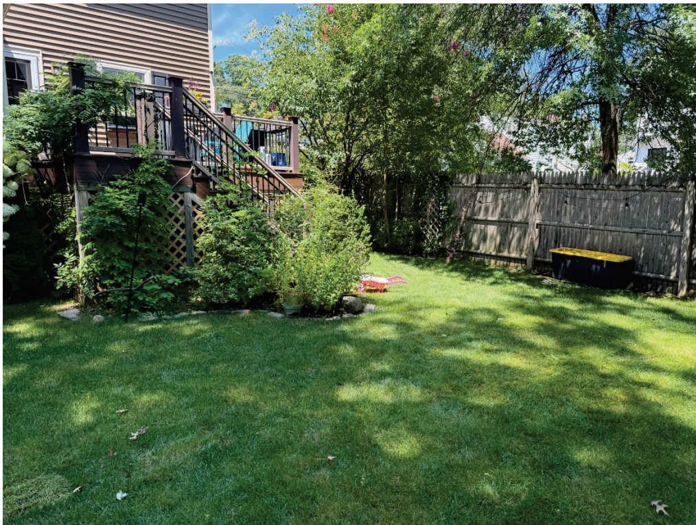
Photo 3 – View of the rear deck, and rear of the dwelling.
